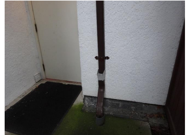
Downspout connection to the underground drain pipe
