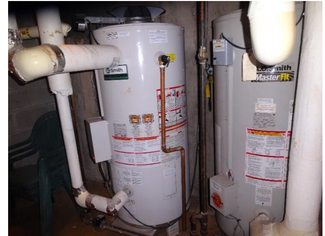
Domestic hot water storage tanks
