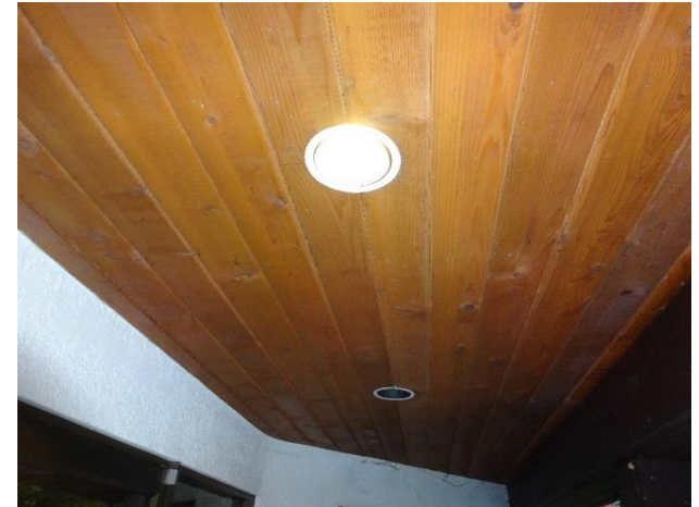
Soffit mounted light fixtures
