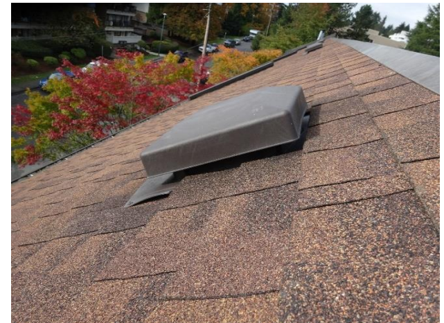
Asphalt shingle roofing system
