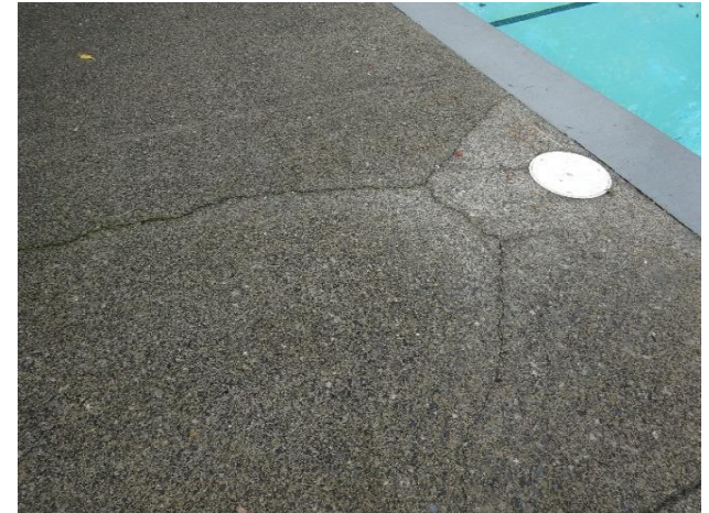
Cracked pool concrete decking
