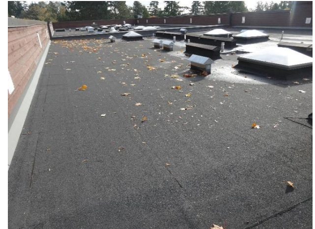
SBS membrane roofing system
