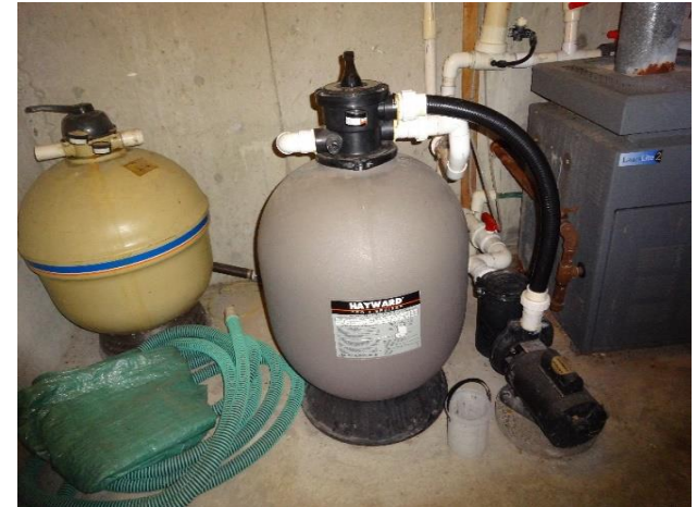
Sand filter, pump and piping
