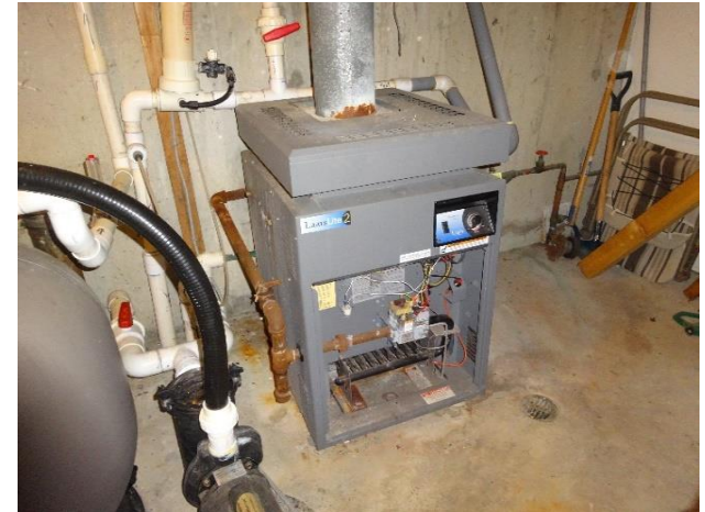
Pool heating boiler
