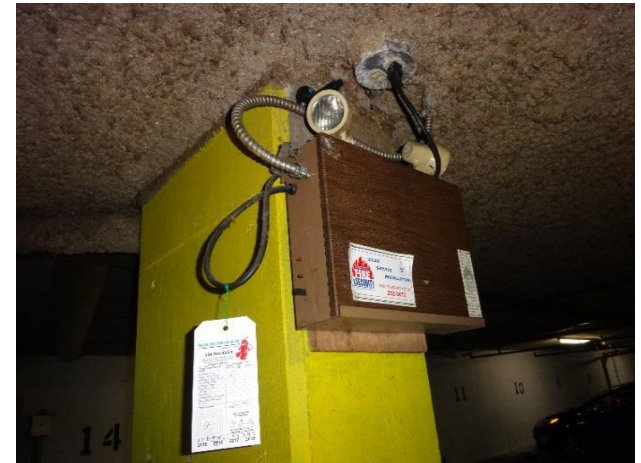
Obsolete emergency lights and battery package
