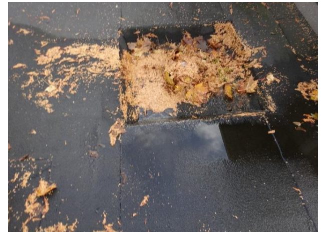
Clogged roof drain
