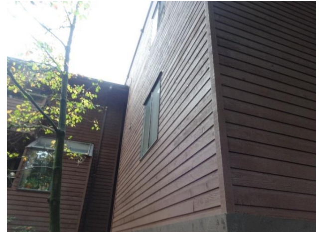
Replaced section of wood cladding
