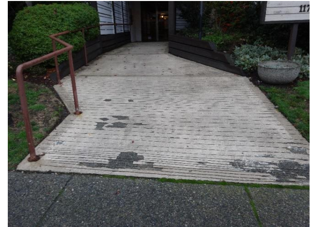
Front walkway with delamination
