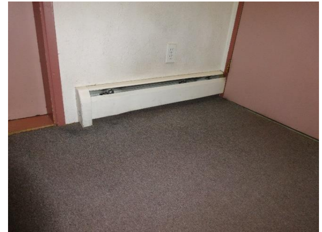
Hot water heating baseboard
