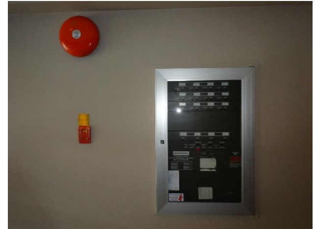
Annunciator panel, alarm bell, pull station
