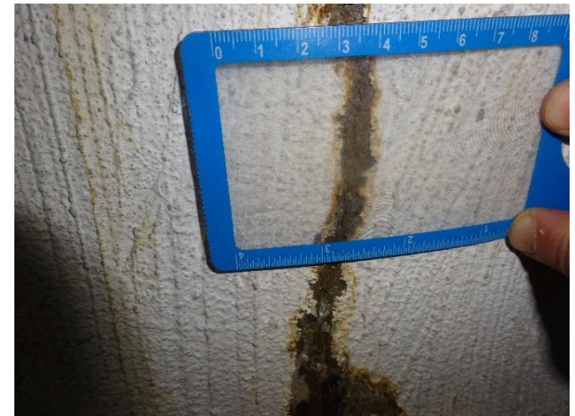
Leaking crack on wall
