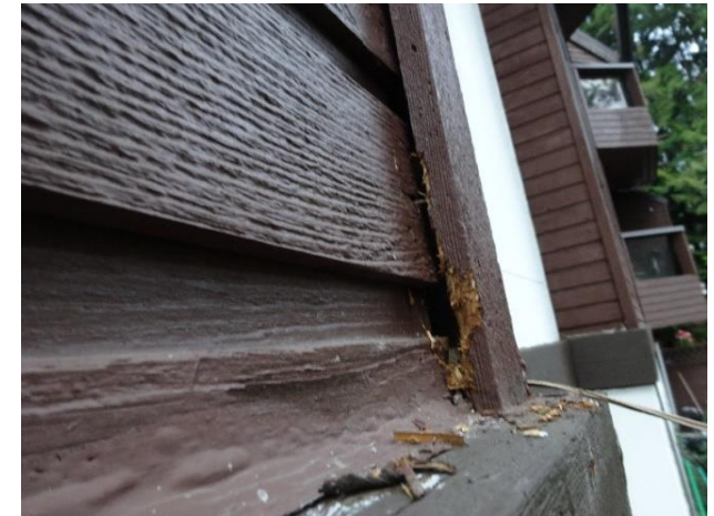
Rotten wood cladding/trim
