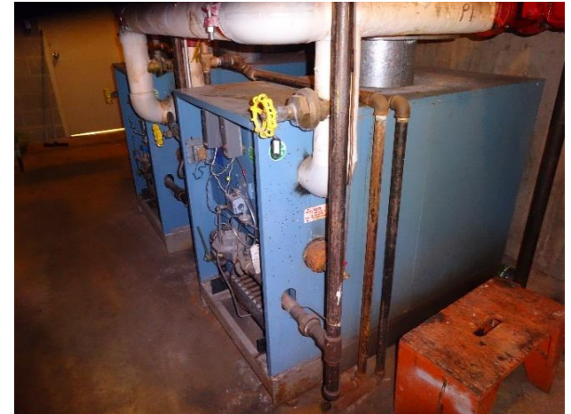
Hot water heating boilers
